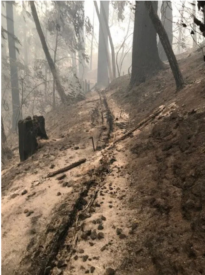
Melted plastic was all that remained Aug. 21, 2020, of a pipeline that supplied the Lyon Water Treatment Plant after the CZU Lightning Complex Fire ravaged the area near Boulder Creek. (San Lorenzo Valley Water District — Contributed)
