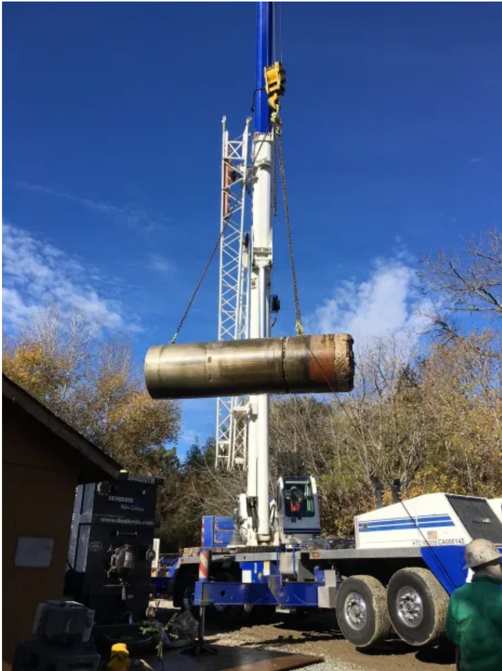
Removal of the micro-tunneling equipment on the east side of the San Lorenzo River. (Contributed photo — City of Santa Cruz Water Department)
