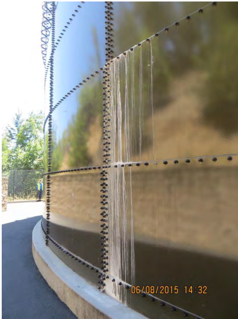
Photo 2-81: Glenwood Tank – Evidence of Past Leakage at Top of Second Shell Course
