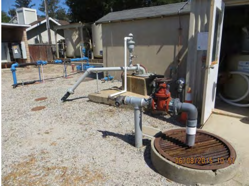
Photo 2-5: Well 9 Mechanical Layout
