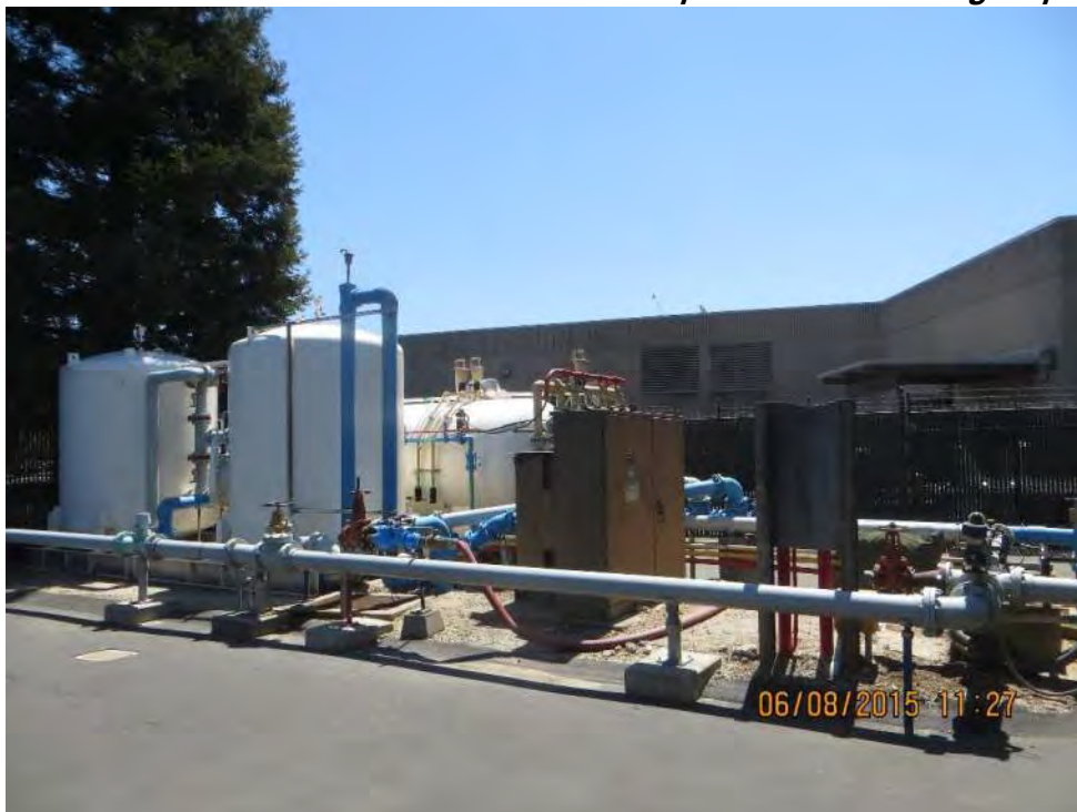
Photo 2-10: Well 10A Exposed PVC Discharge Pipe
