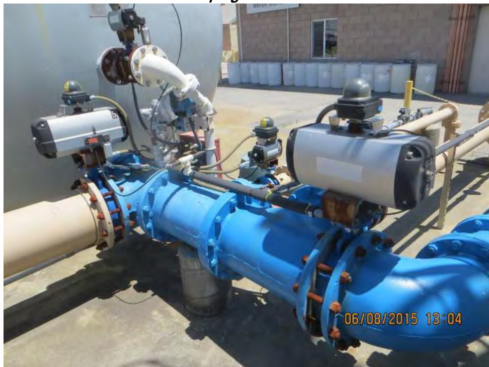
Photo 2-28: El Pueblo Water Treatment Plant Yard Piping with Corrosion on All-Thread & Bolts
