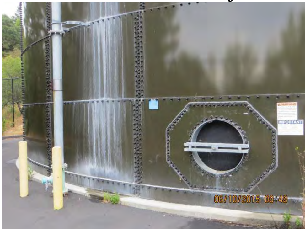
Photo 2-110: Recycled Water Tank – Make-Up Water Staining on Tank Exterior
