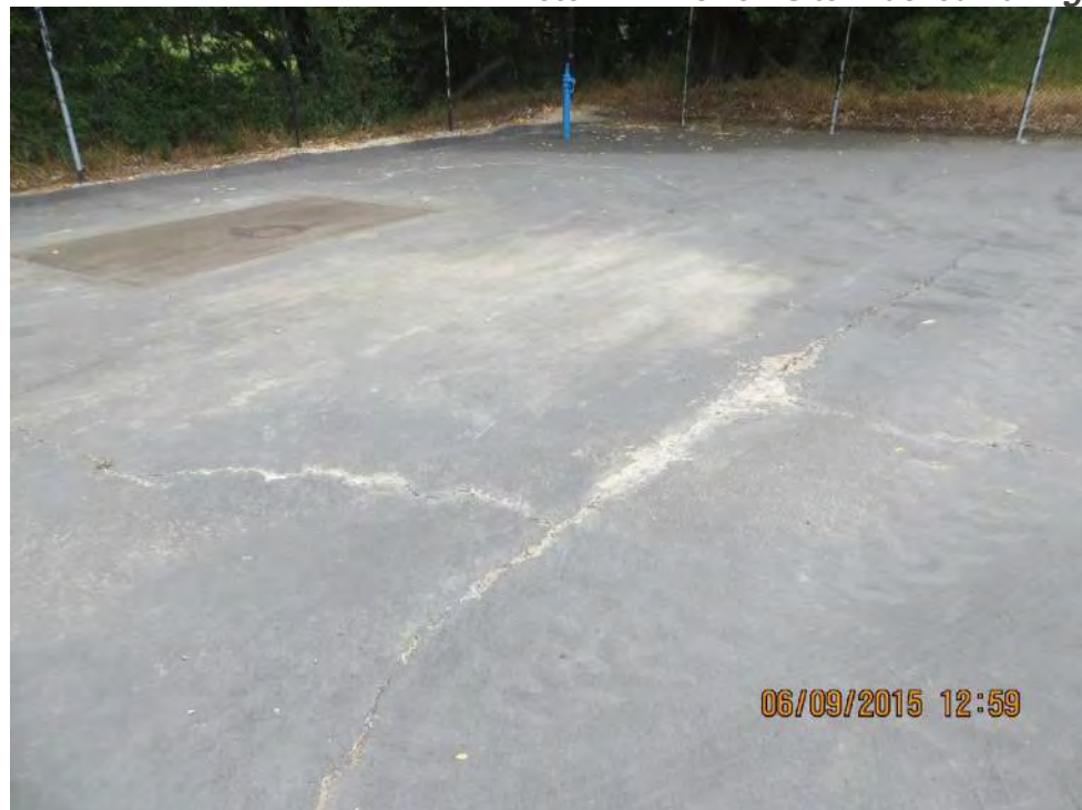
Photo 2-2: Well 3B Site Cracked Paving
