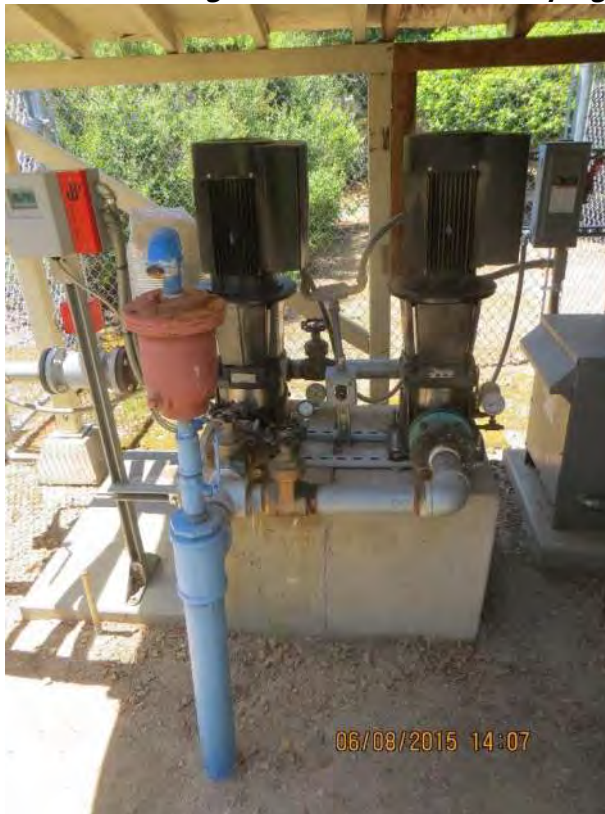
Photo 2-55: Hacienda Pump Station – Unpainted Timber in Background & Corrosion on Piping
