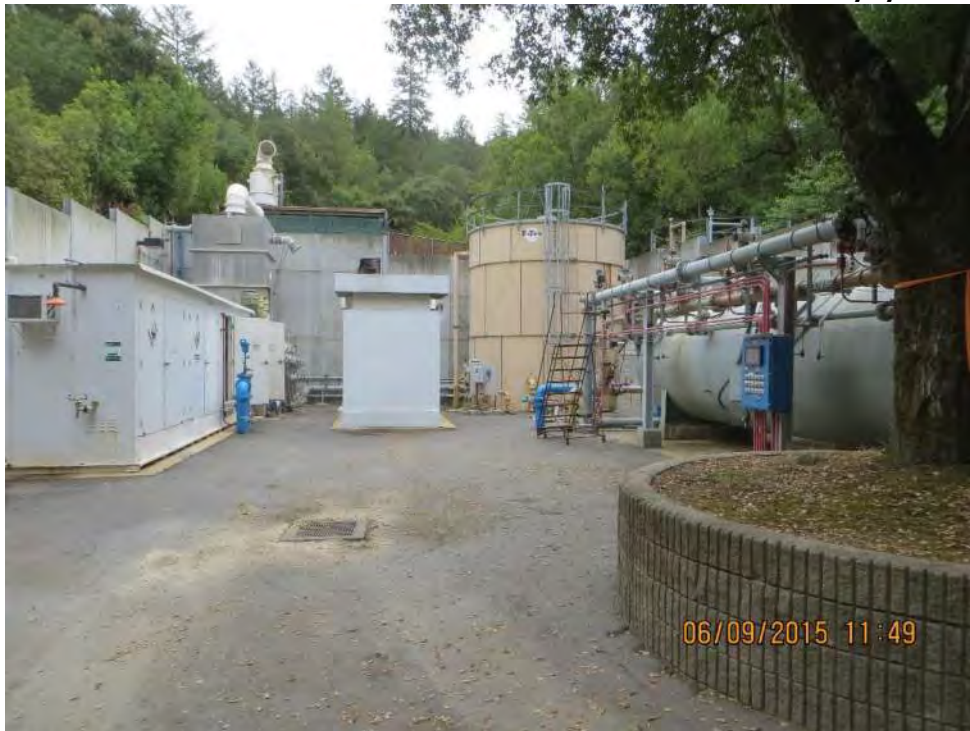
Photo 2-30: Orchard Run Water Treatment Plant Dual Media Pressure Filter and Treatment Equipment
