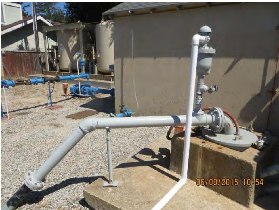
Photo 2-6: Well 9 Mechanical – Minor Corrosion & No Check Valve
