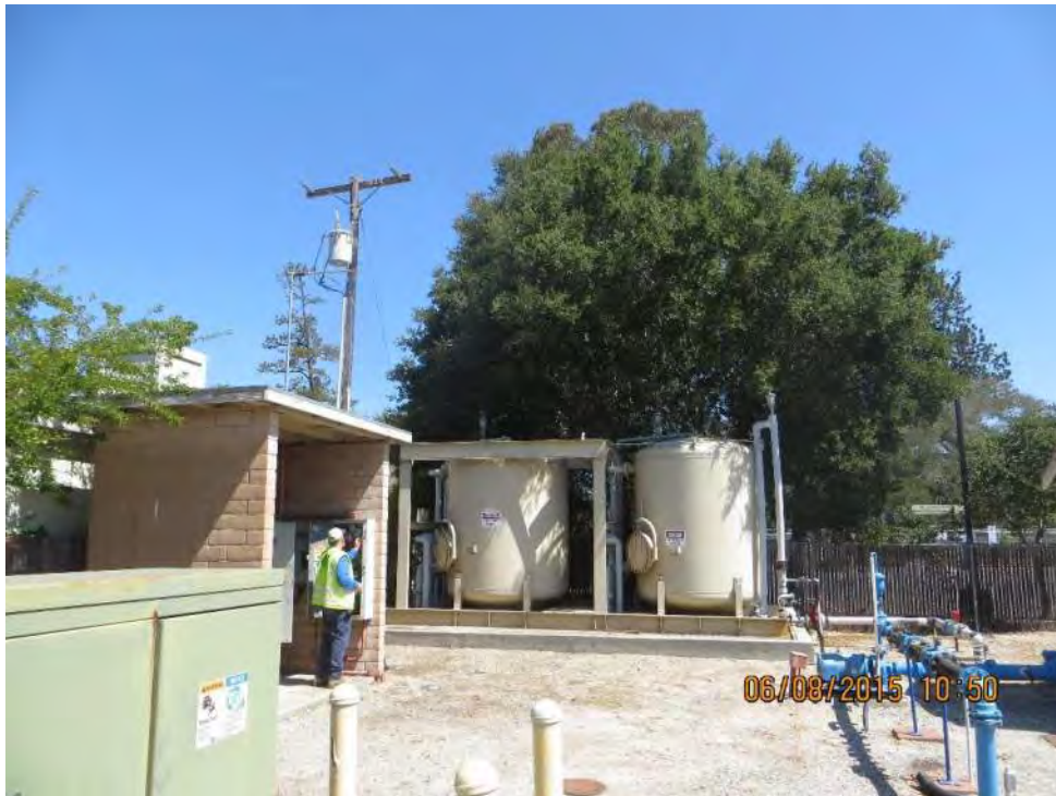
Photo 2-15: Well 9 Water Treatment Plant GAC Pressure Filters and Electrical Gear
