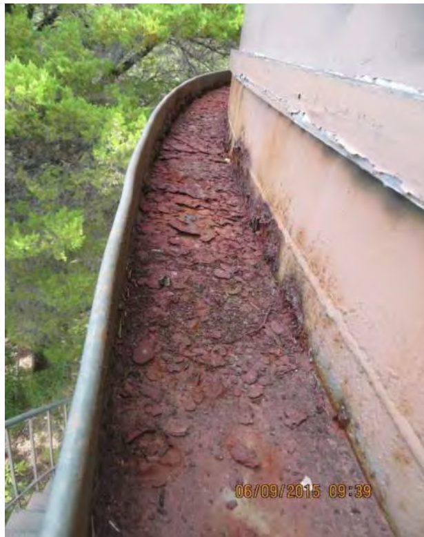
Photo 2-72: Bethany Tank – Corrosion at Gutter/Top Shell Course
