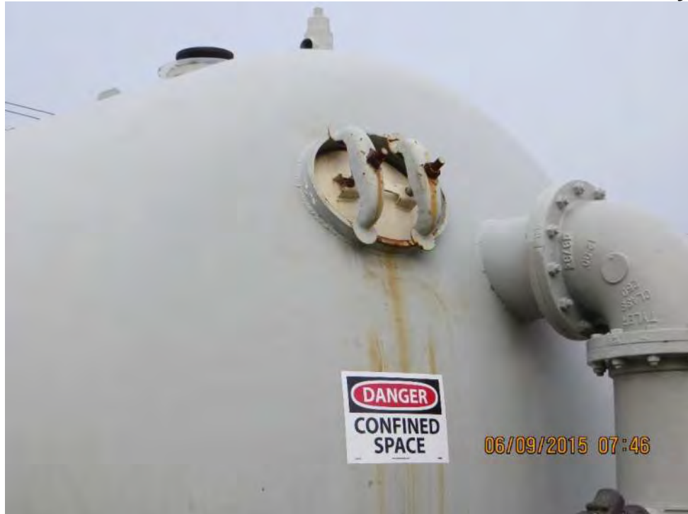
Photo 2-28: El Pueblo Water Treatment Plant Yard Piping with Corrosion on All-Thread & Bolts
