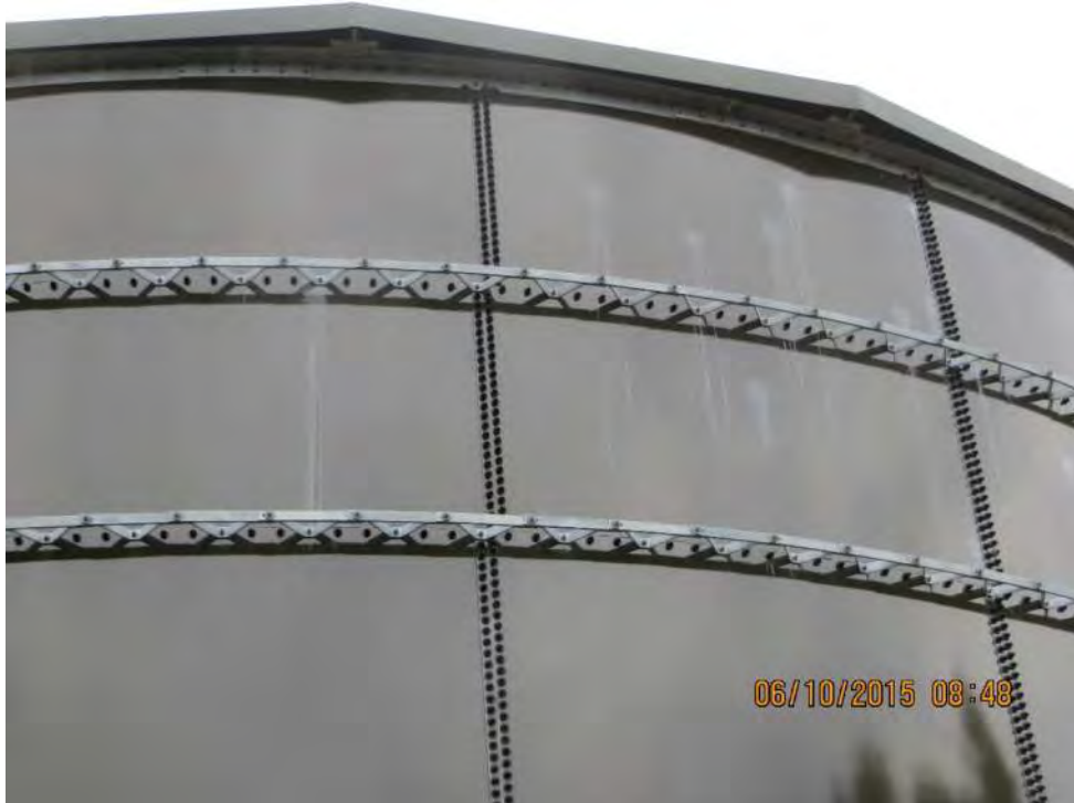
Photo 2-109: Recycled Water Tank – Marring of Tank Exterior Coating from Paintballs
