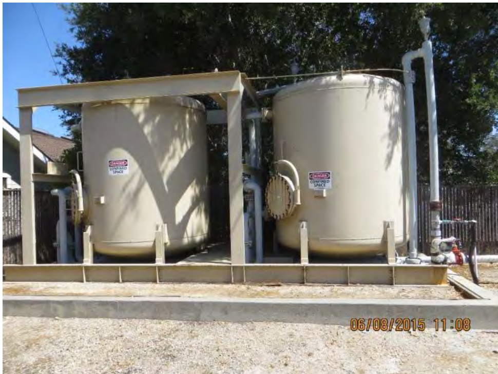
Photo 2-17: Well 9 Water Treatment Plant GAC Pressure Filters
