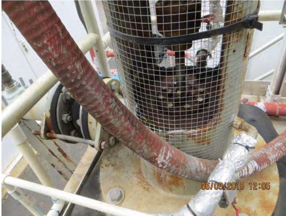
Photo 2-66: Orchard Run WTP Pump Station Leaking Mechanical Seal and Corrosion
