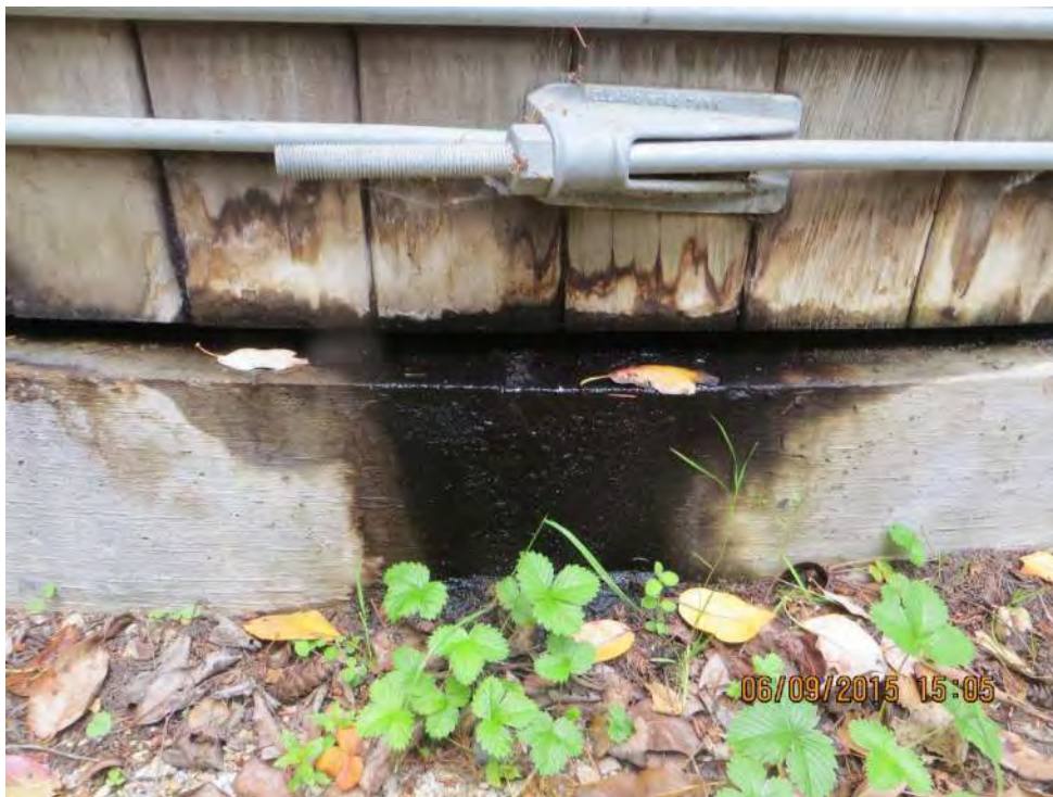
Photo 2-101: Villa Fonteney Tank – External Tank Leakage at Tank Base
