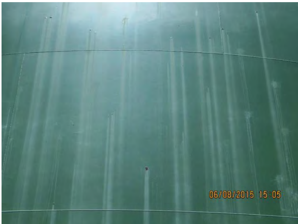
Photo 2-93: Sequoia Tank - Paintball Marring & Corrosion on Exterior of Tank
