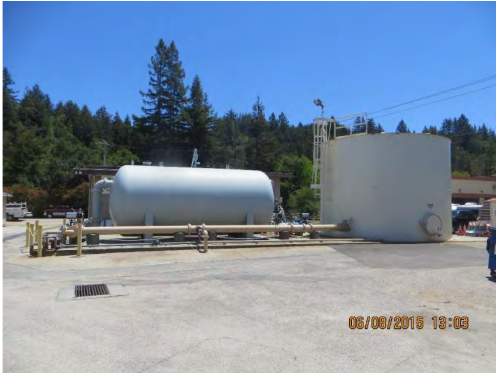
Photo 2-23: El Pueblo Water Treatment Plant Dual Media Pressure Filter & Backwash Tank
