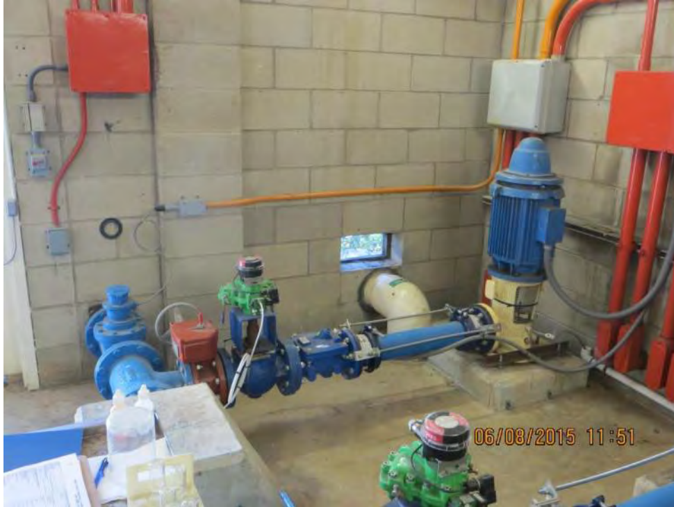
Photo 2-60: Well 10A WTP Pump Station Discharge Configuration
