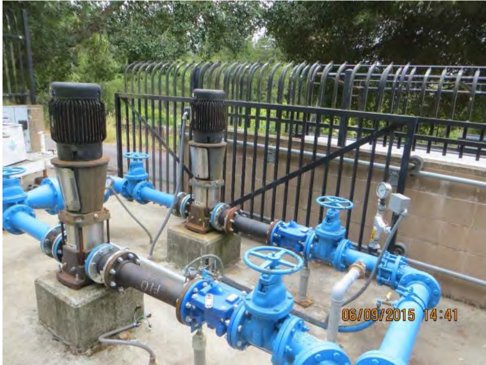
Photo 2-41: Crescent Pump Station Site and Uncoated Sections of Ductile Iron Pipe
