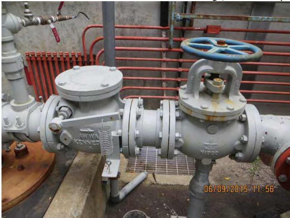
Photo 2-4: Well 7A Corrosion on Well Head Flange, Valves and Pipe
