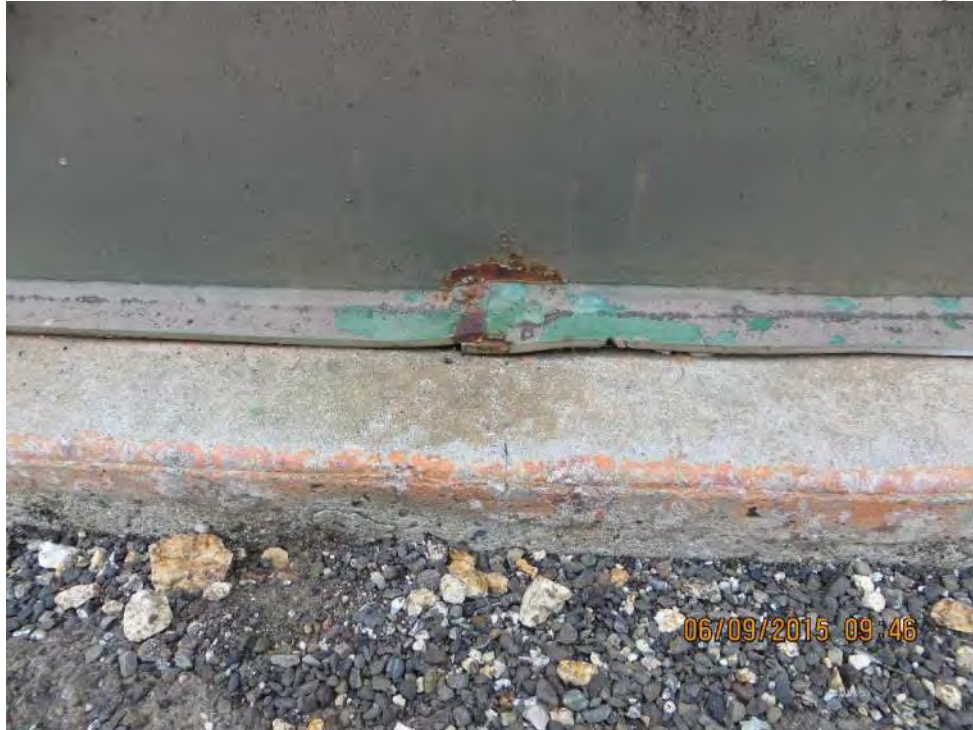
Photo 2-73: Bethany Tank – Corrosion at Base Flange
