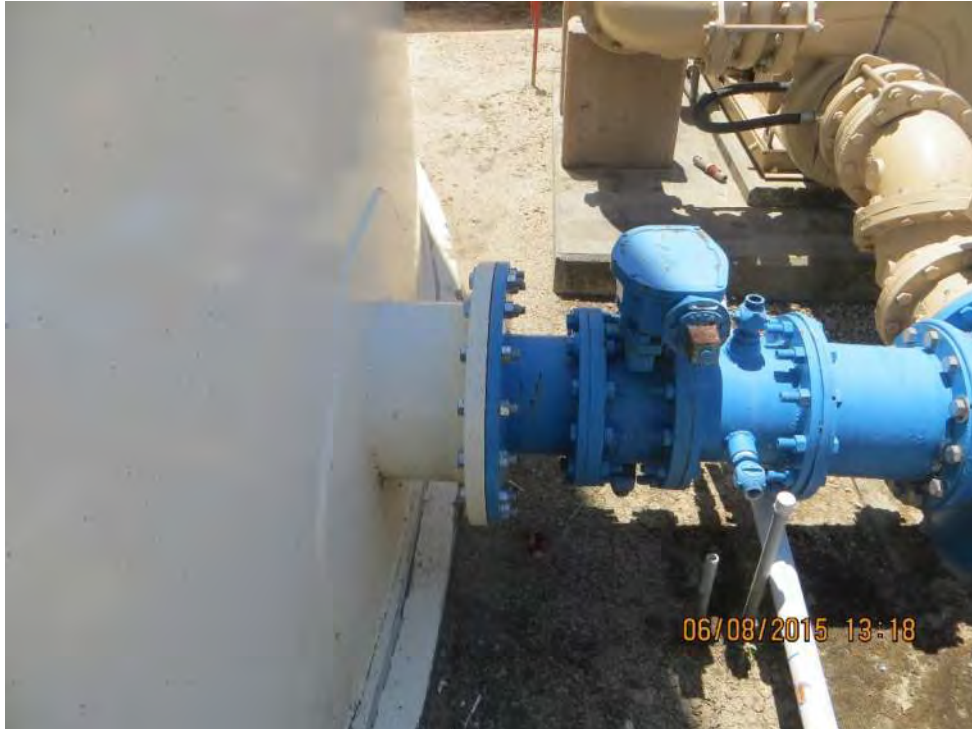
Photo 2-79: El Pueblo Tank – Area of Potential Ponding (Ground Flush with Ring Wall Footing)
