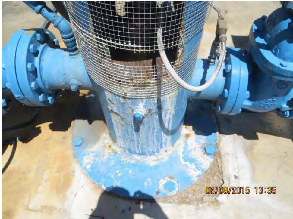
Photo 2-63: El Pueblo WTP Pump Station Leaking Mechanical Seal and Corrosion
