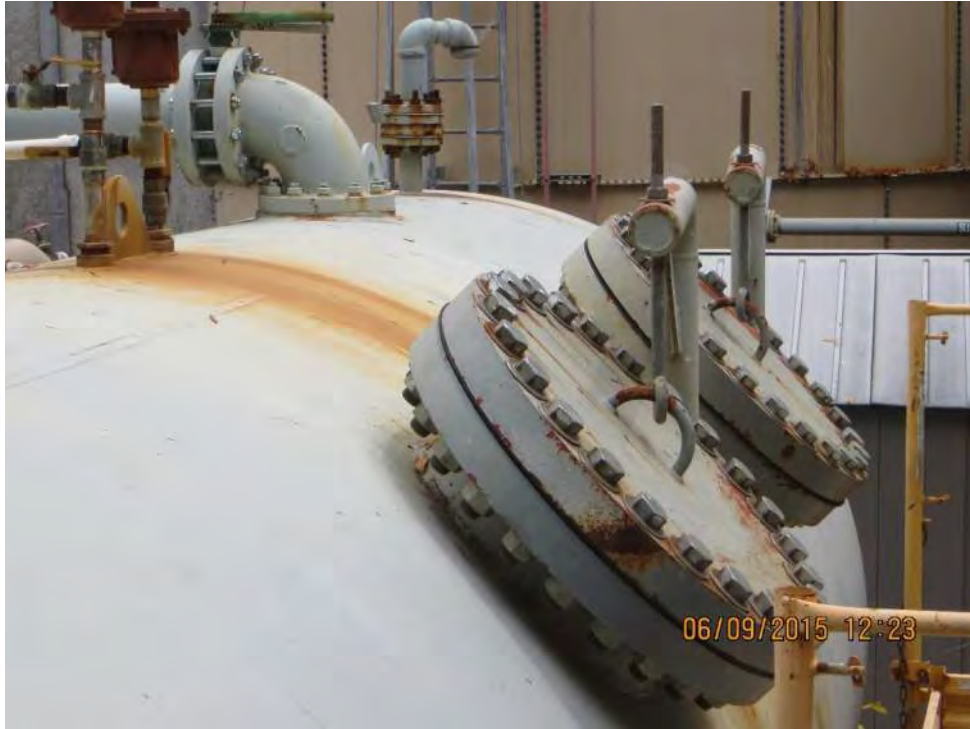
Photo 2-37: Orchard Run Water Treatment Plant Dual Media Pressure Filter (External Corrosion)
