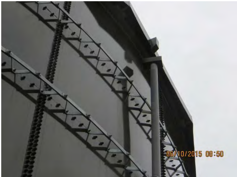
Photo 2-108: Recycled Water Tank – Roof Drain Detached from Gutter System
