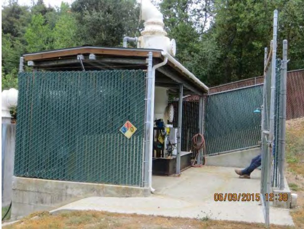
Photo 2-31: Orchard Run Water Treatment Plant Flume Scrubber
