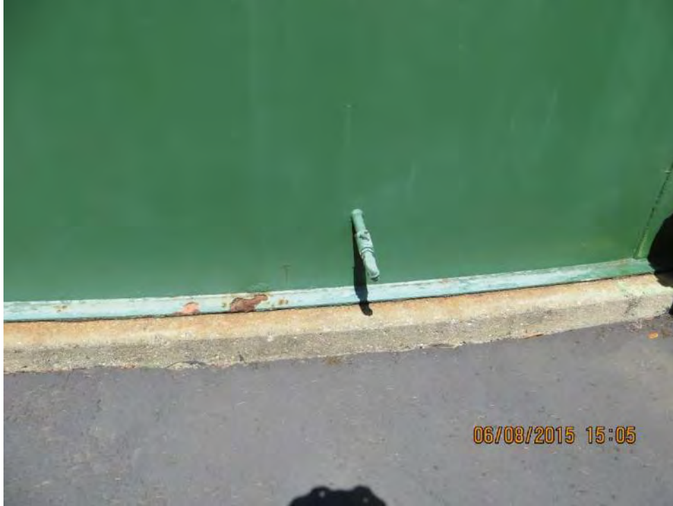
Corrosion at Tank Base Flange
