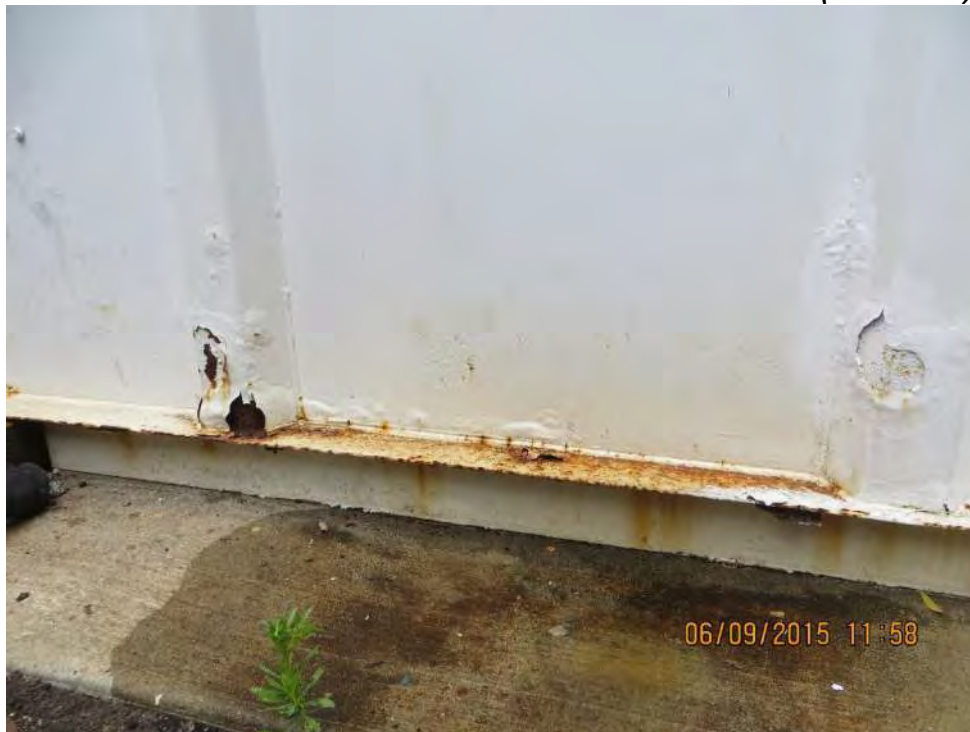
Photo 2-34: Orchard Run Water Treatment Plant Chemical Feed Building (Corrosion)
