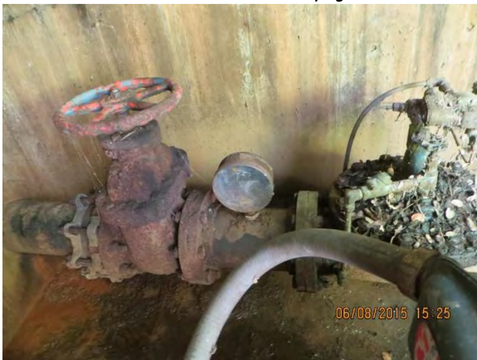
Photo 2-51: Southwood Pump Station – Corrosion of Valve and Piping & Debris on Cla-Val
