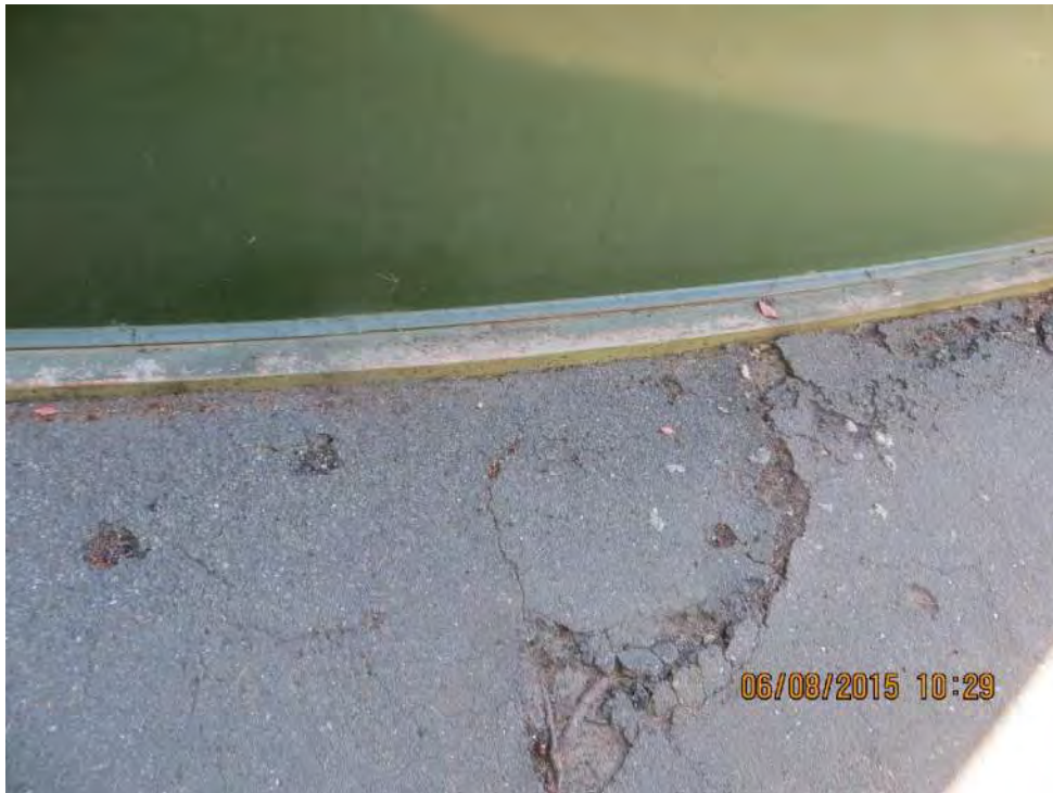
Photo 2-87: Macdorsa Tank – Root Intrusion
