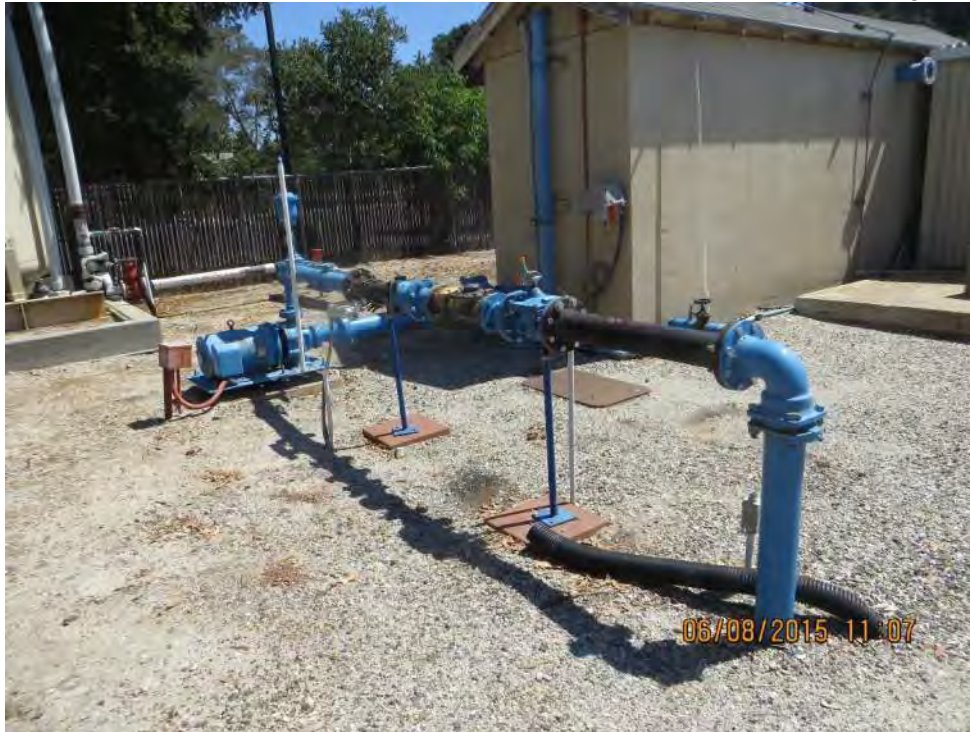
Photo 2-56: Well 9 WTP Booster Pump Mechanical Layout
