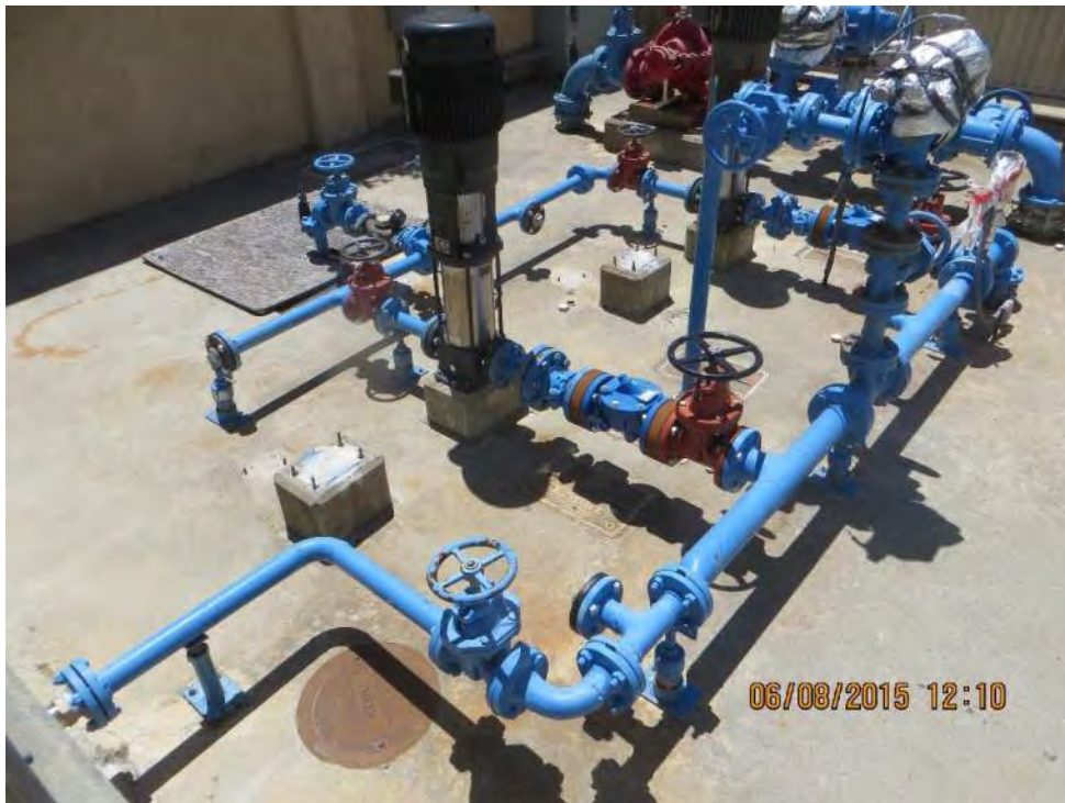
Photo 2-53: Monte Fiore Pump Station – Uncoated Flanges and Areas of Minor Corrosion
