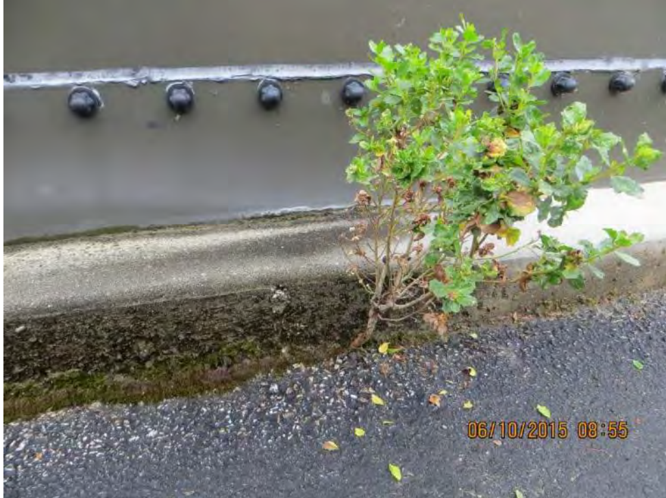
Photo 2-111: Recycled Water Tank - Vegetation Growing at Tank Ring Wall Footing
