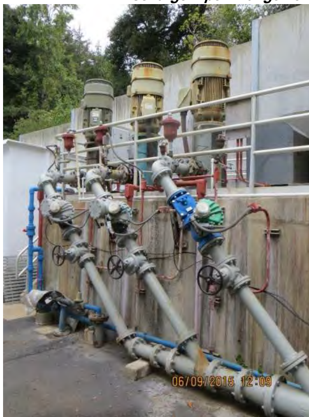
Photo 2-65: Orchard Run WTP Pump Station Discharge Pipe Arrangement
