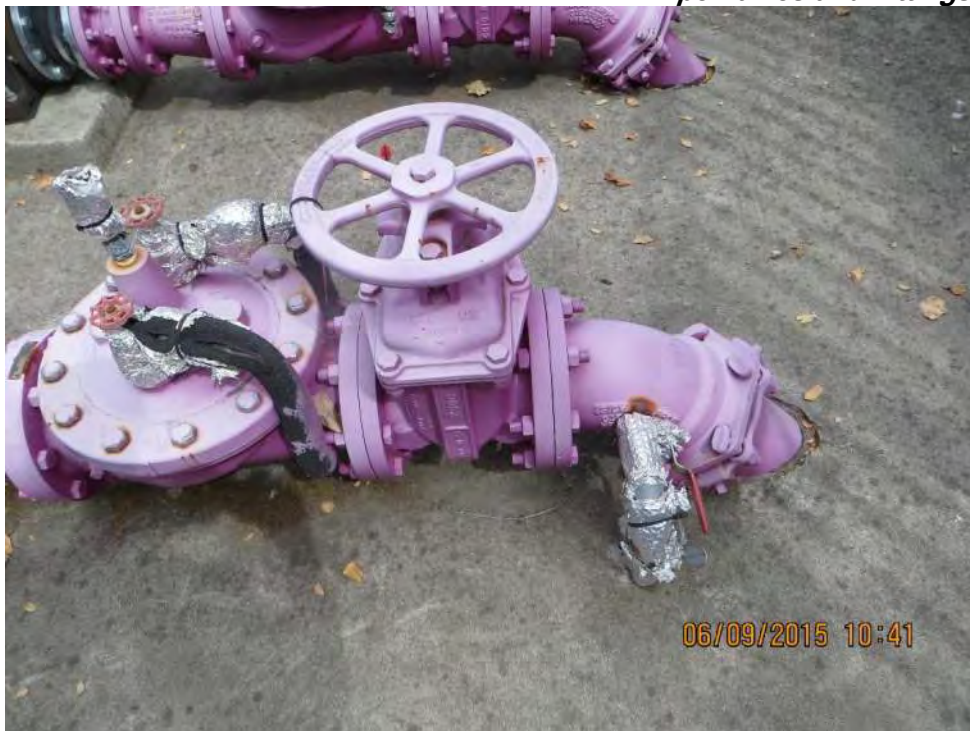
Photo 2-105: Siltanen Pump Station – Corrosion on Pipe Valves and Fittings
