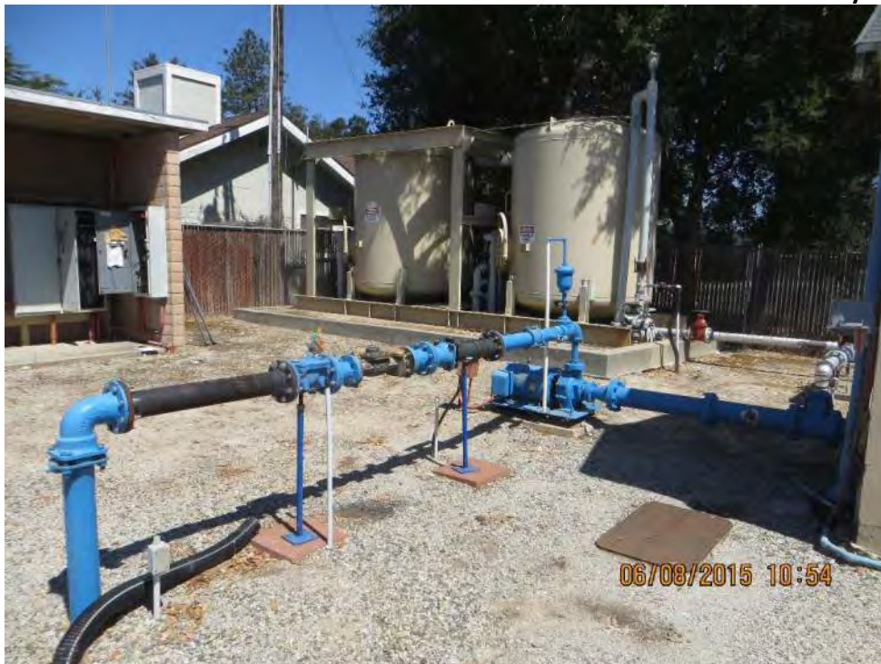
Photo 2-57: Well 9 WTP Booster Pump Uncoated Sections of Ductile Iron Pipe
