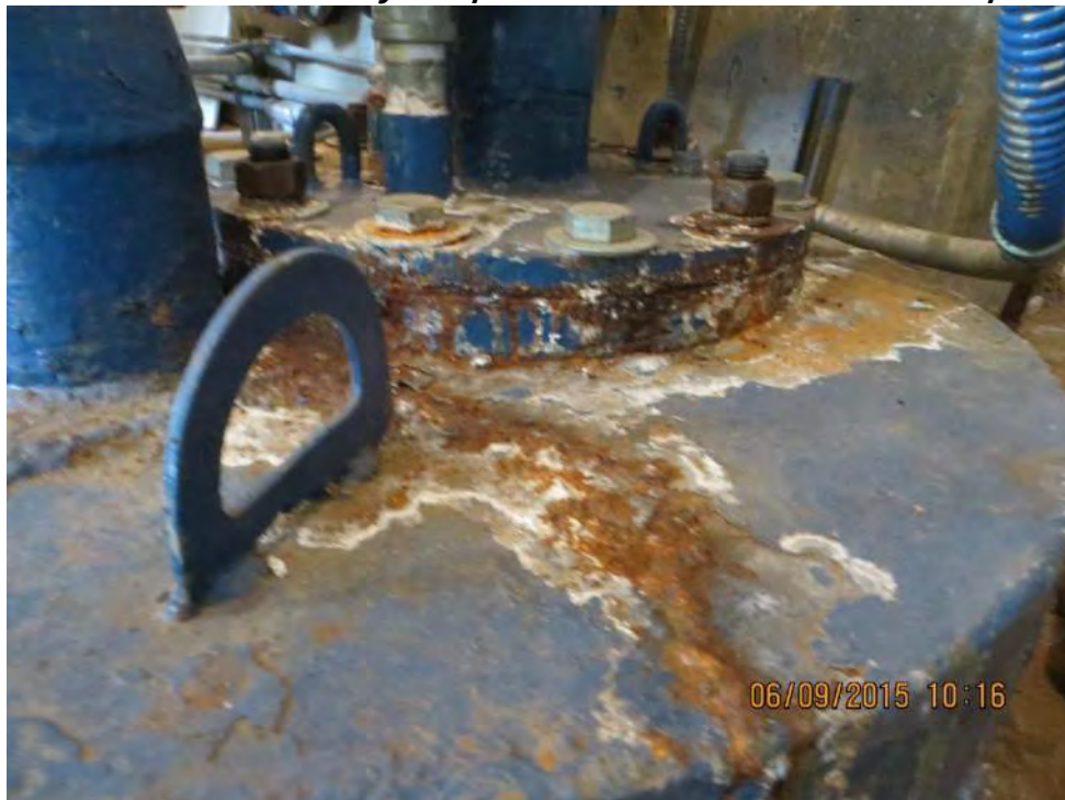
Photo 2-45: Bethany Pump Station Corrosion on Sealed Pump Can
