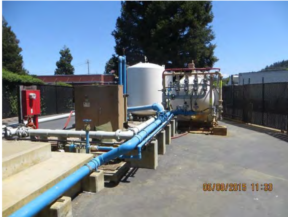
Photo 2-19: Well 10A Water Treatment Plant Dual Media Pressure Filter, GAC Filters, Exposed PVC Pipe
