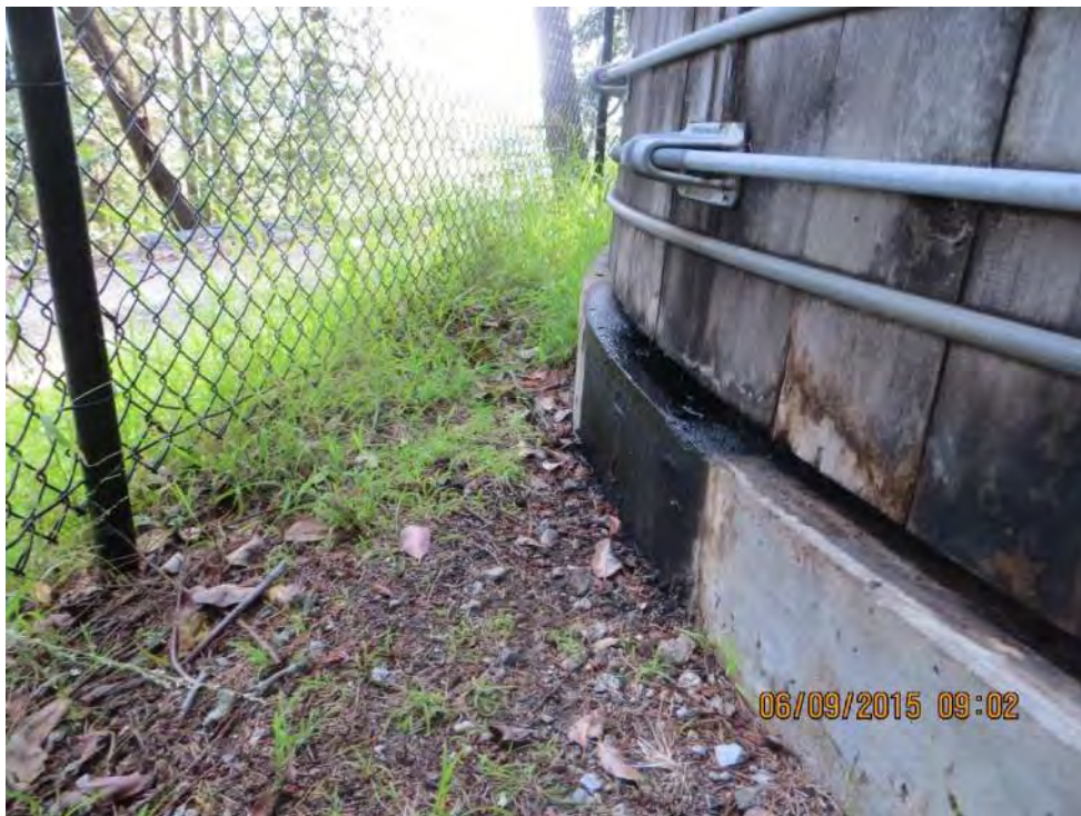
Photo 2-89: Mt. Roberta Tank – Leakage at Tank Base
