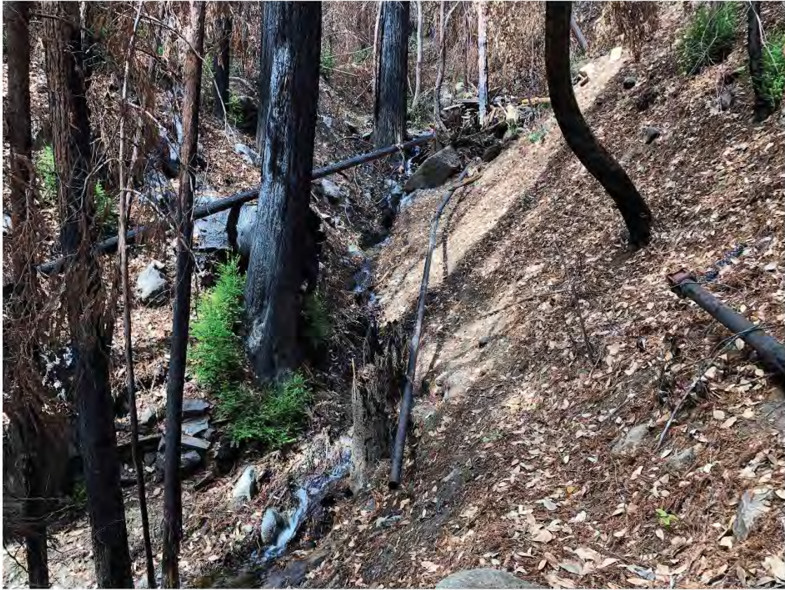
Typical fire damage in the watersheds.
