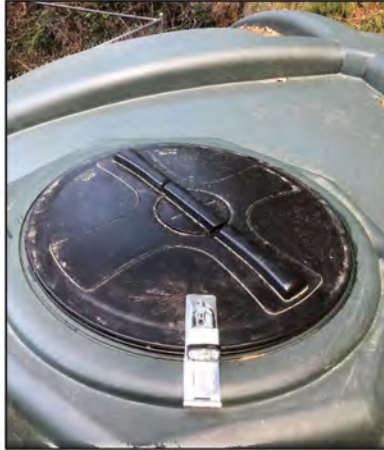
Figure 10: Roof lock on China Grade Tank.
