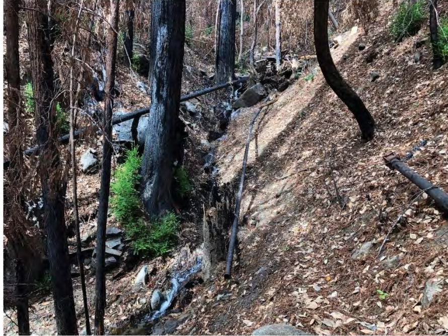
Corvin Creek intake not yet repaired.
