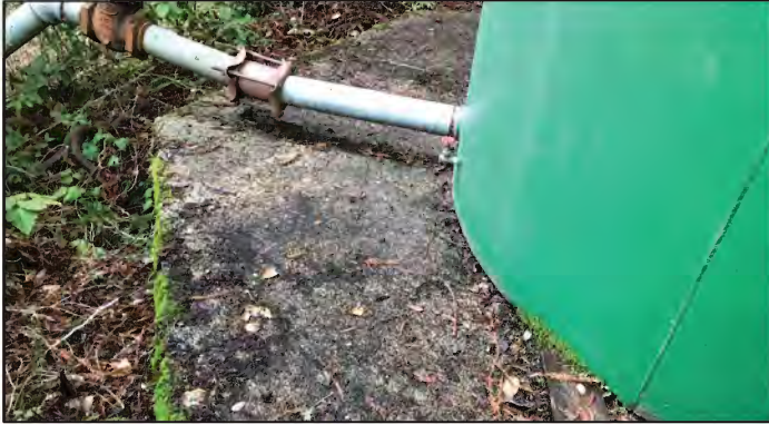
Figure 12: Oberst Station existing foundation
