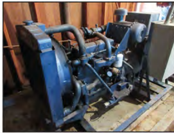
Figure 9. Generator repaired and operational
