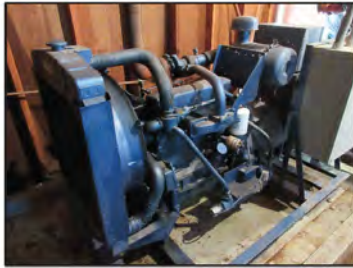
Figure 9. Generator repaired and operational
