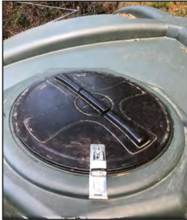
Figure 10: Roof lock on China Grade Tank.
