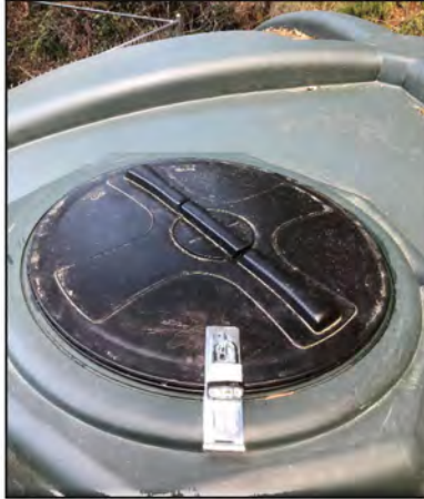
Figure 10: Roof lock on China Grade Tank.
