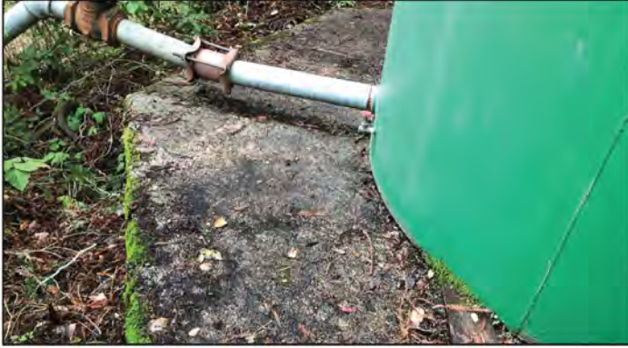
Figure 12: Oberst Station existing foundation
