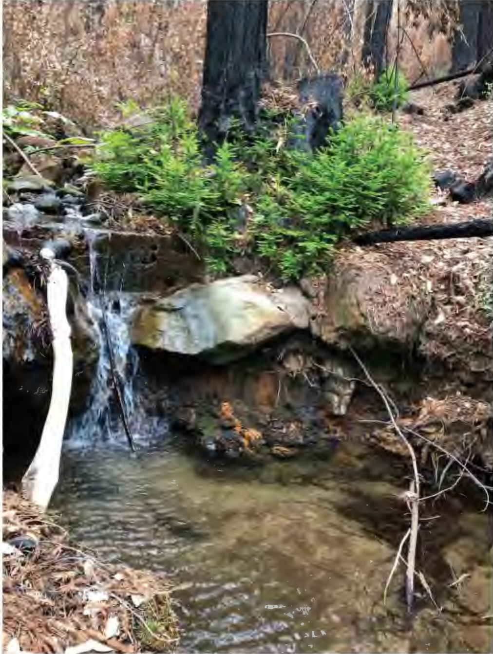
North Creek intake prior to repairs completed in summer 2021.
