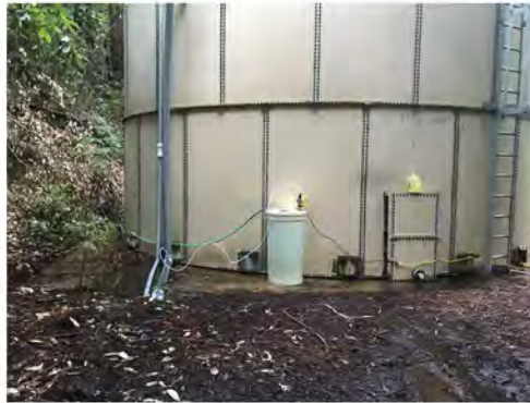
Figure 1. Temporary Disinfectant Injection Configuration at Well # 4
