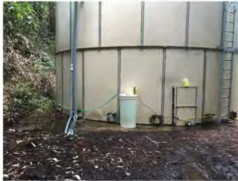
Figure 1. Temporary Disinfectant Injection Configuration at Well # 4
