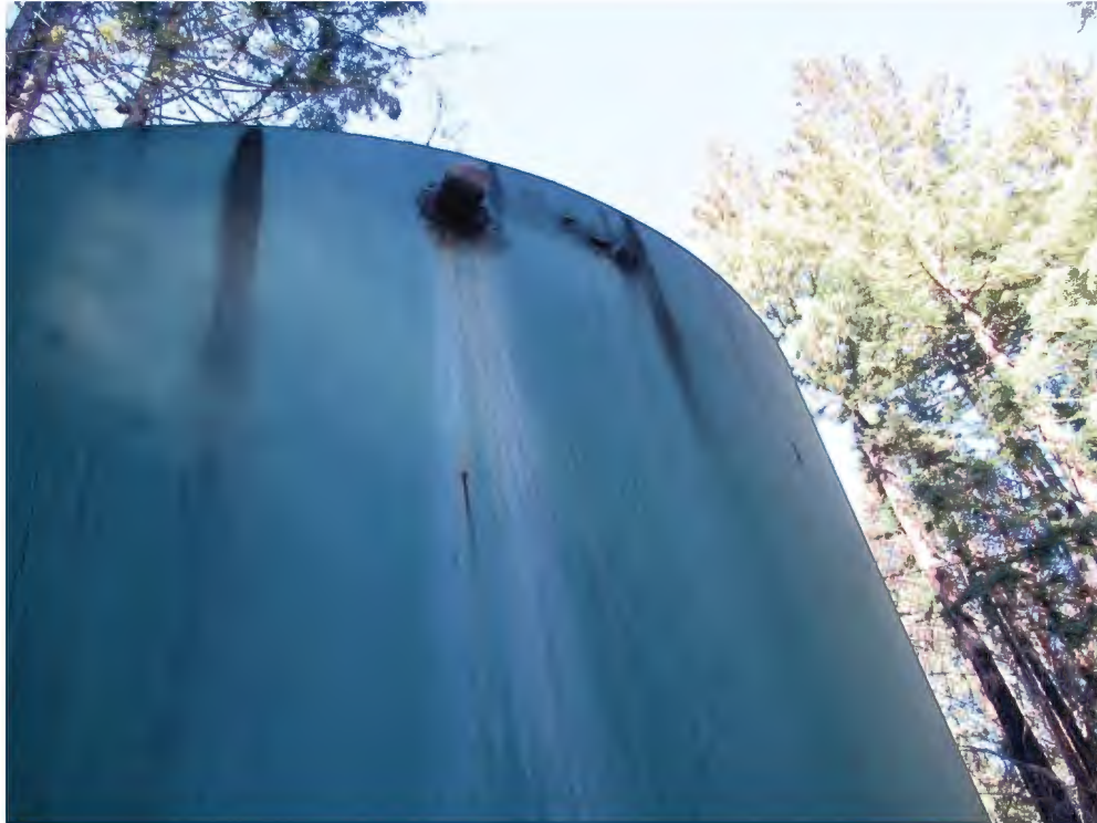
Holes in the Tank Sidewall
