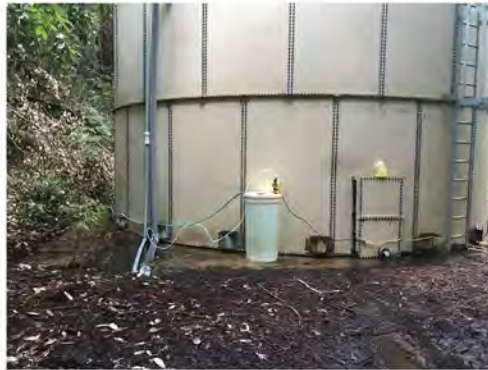
Figure 1. Temporary Disinfectant Injection Configuration at Well # 4
