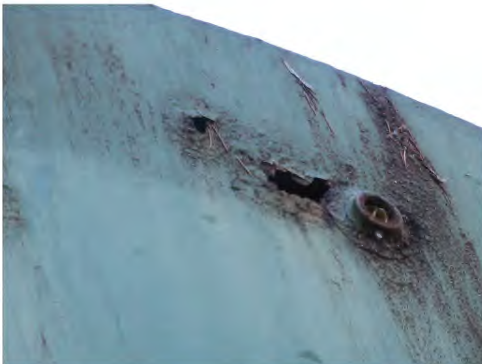
Enlarged Image of Tank Sidewall Holes
