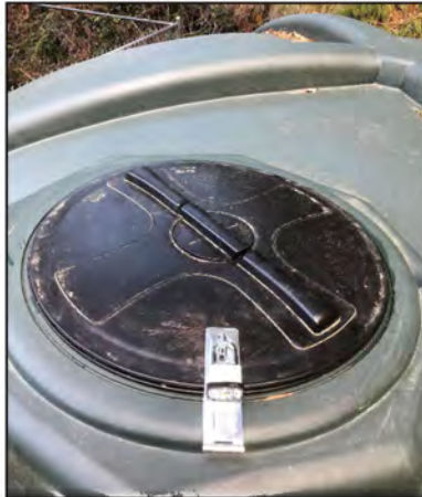
Figure 10: Roof lock on China Grade Tank.
