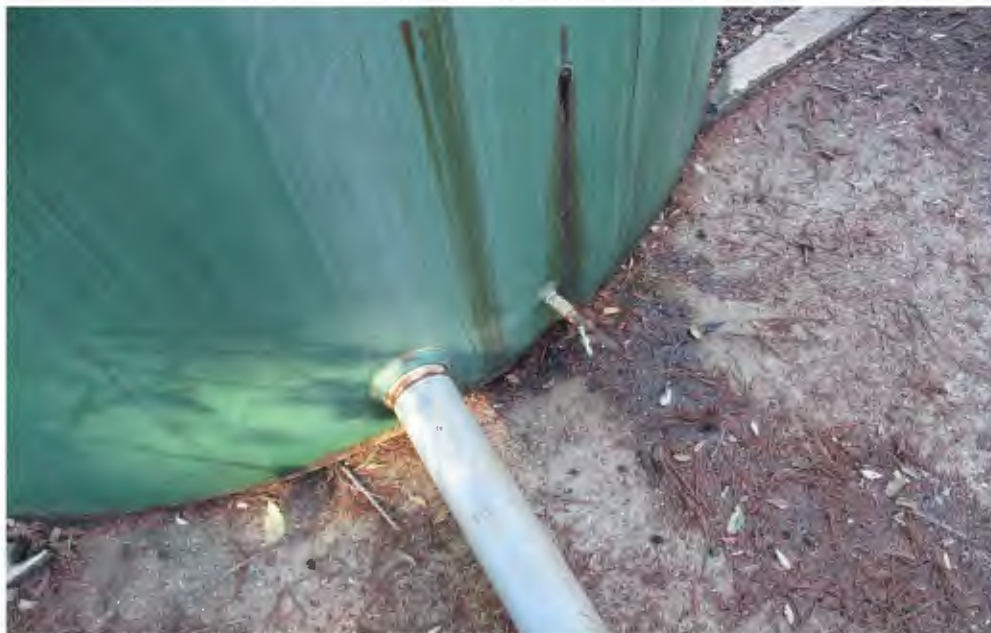
Corrosion and Leaks in the Tank Sidewall
