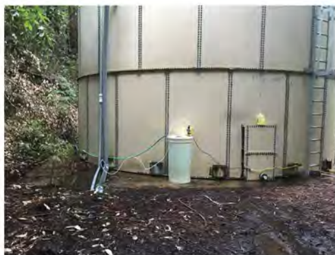
Figure 1. Temporary Disinfectant Injection Configuration at Well # 4
