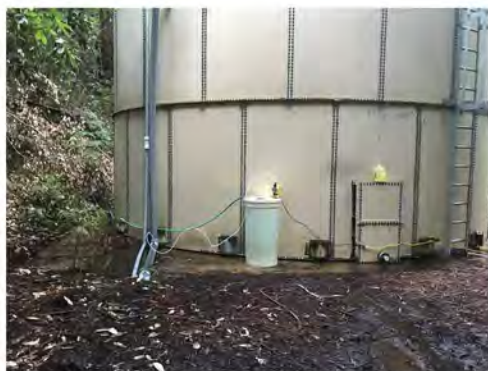
Figure 1. Temporary Disinfectant Injection Configuration at Well # 4
