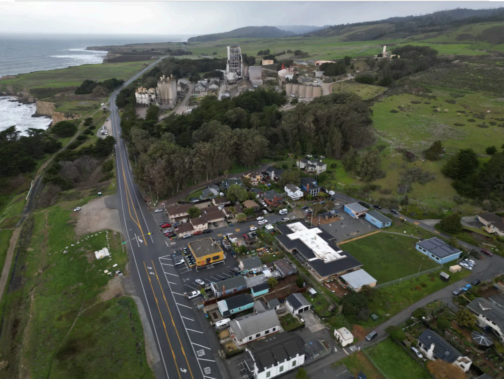
An aerial view of the town of Davenport and the Cemex cement plant. Credit: Kevin Painchaud / Lookout Santa Cruz
